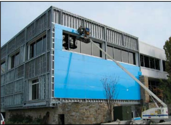
*Welded Steel tube system has been installed and supported at the base. Cold formed metal stud framing and new facade installation is in progress.*
