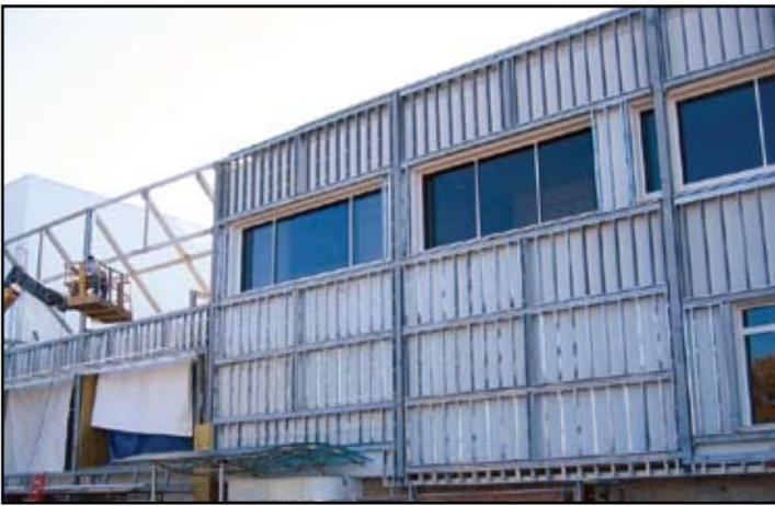
*In order to resist the wind loads the front entrance welded steel tube framing had to be braced back diagonally to the existing roof framing.*
